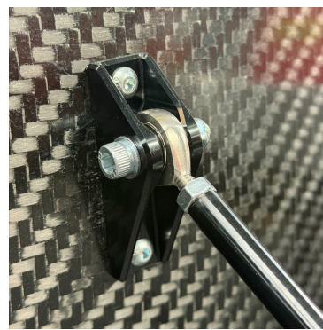
Rod end adjustment
